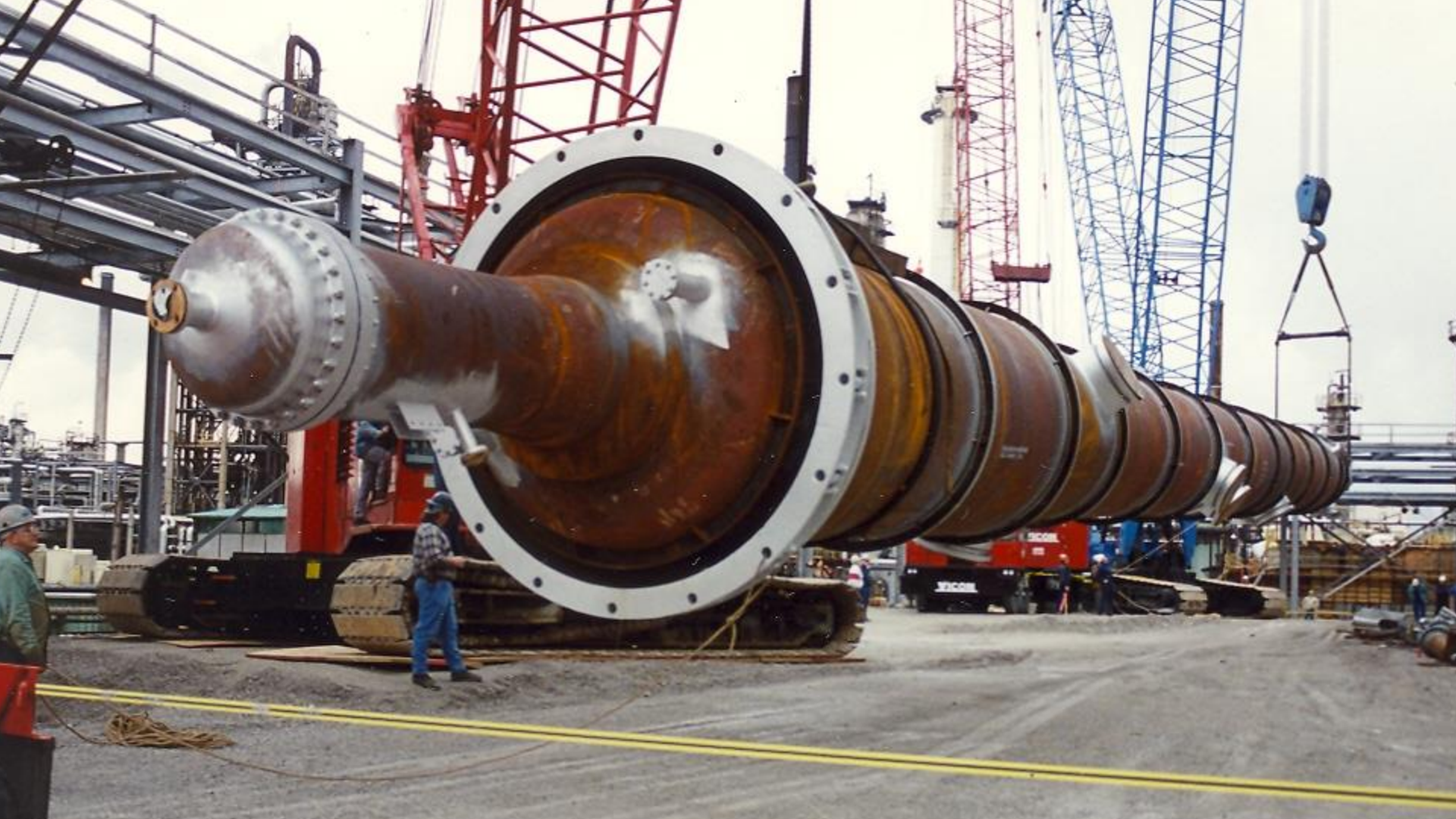
Lowboy pulled forward through pipe rack Steerable dolly rolled out backward
